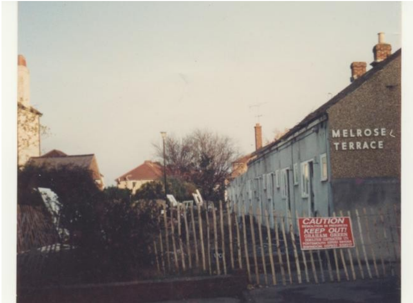
Fig 15 – Melrose Terrace Almshouses in 1992 awaiting demolition.
